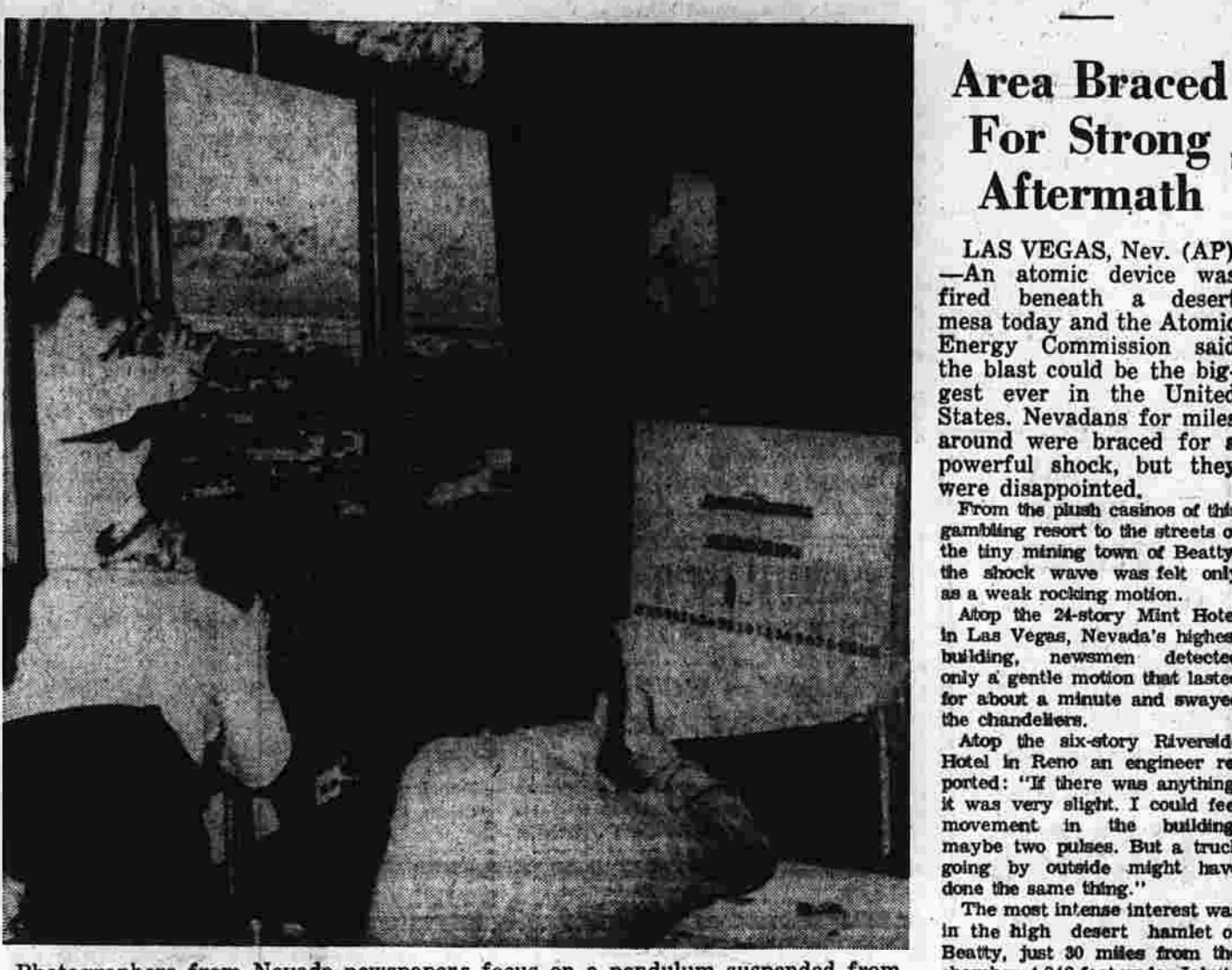
Photographers from Nevada newspapers focus on a pendulum suspended from the Sky Room of Las Vegas' Mint Hotel to measure tremor caused by huge underground atomic explosion. The top of the 36-story building wavered 36 inches, an engineer said, but the pendulum moved only about one and one-half inches. (AP Photos)
